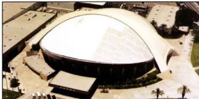
CONVENTION CENTER (metal roof)
